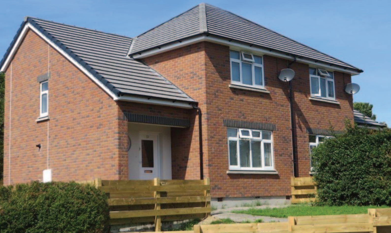
Recently completed externally refurbished houses, Willaston
