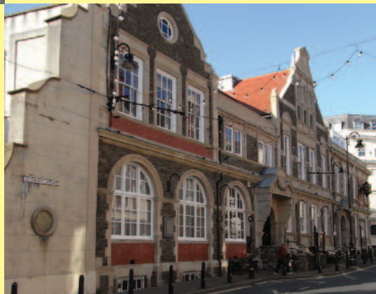
Town Hall following restoration work summer 2009
